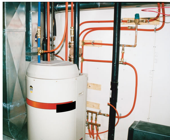
Kitec in mechanical room
